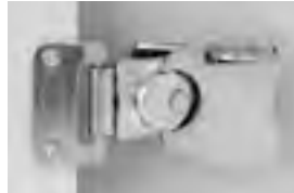
Twist Latch Detail
