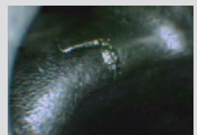
Casting pipe joint
